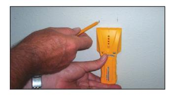
**3.** Using a stud finder, locate the studs in your wall. They should be on 16" centers. We have drilled the holes in the back plate of the wall of the Gun Locker on 16" centers to match the stud placements. Take the measurement from #1 and add 3/4" and mark this on the wall. This is where the top of the Gun Locker will line up.
