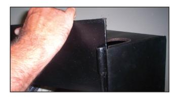
**5.** Using a 3/8" drill bit, pre-drill each hole into the stud at the depth of approximately 4", the depth of the screws. This may prevent stud splitting. If you are installing in a closet end, there should be a double corner stud. Pre-drill at an angle. Always try to center the stud.
